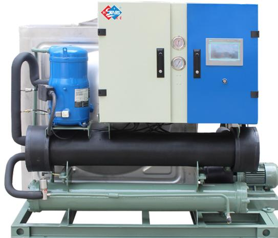
Water-cooled scroll type combined dual-function heating and cooling chiller
